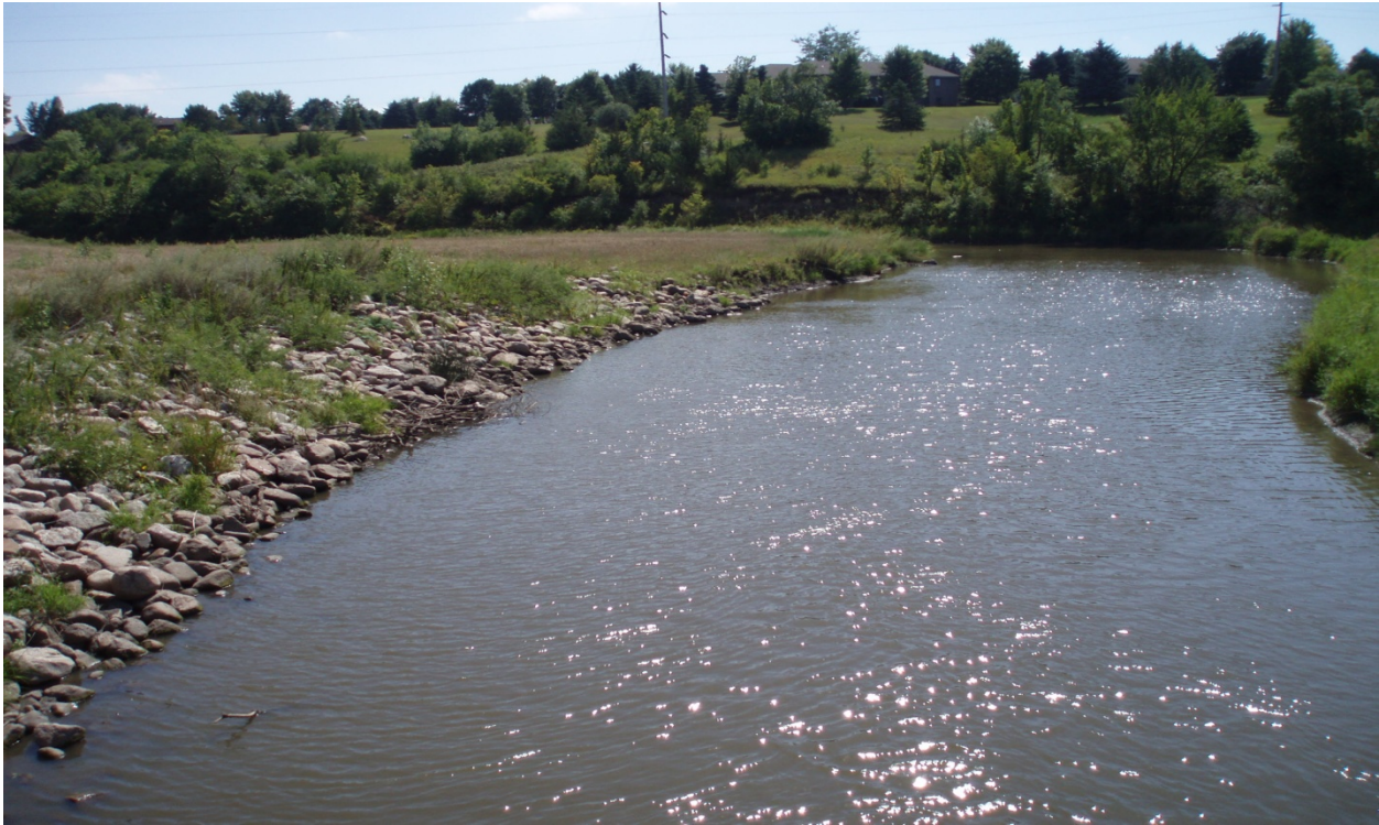
Figure 12: Skunk Creek bank stabilization.
