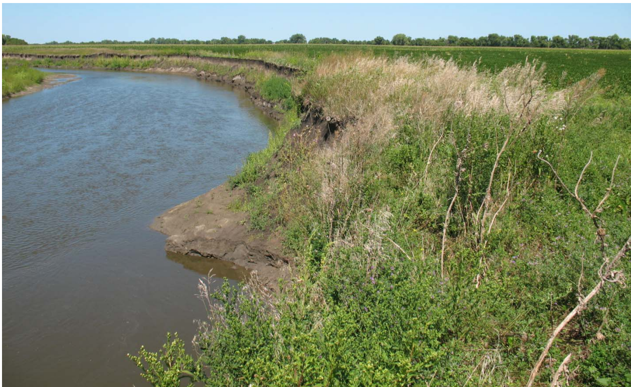
Figure 14: Preconstruction of segment 65.
