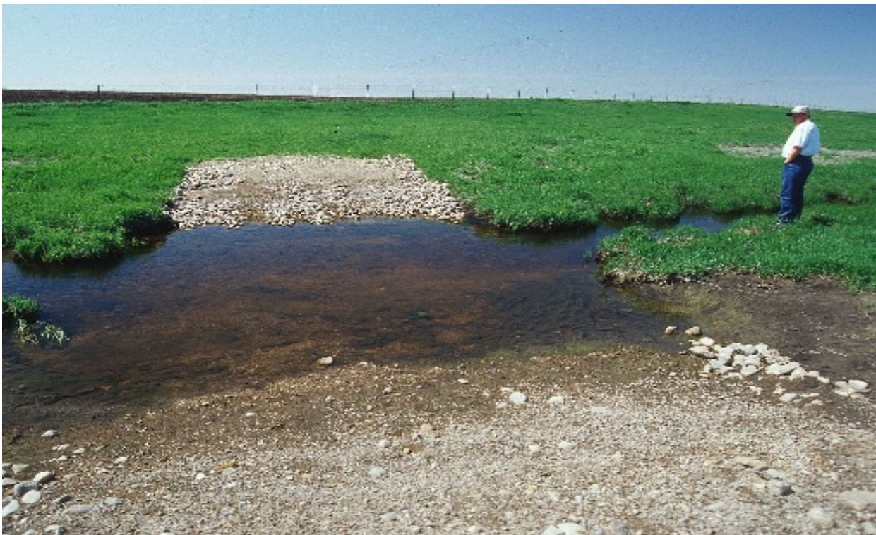
Figure 10: Installed cattle rock crossing.
