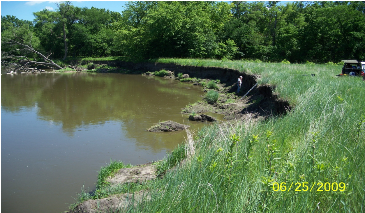
Figure 18: The preconstruction picture of segment 1.
