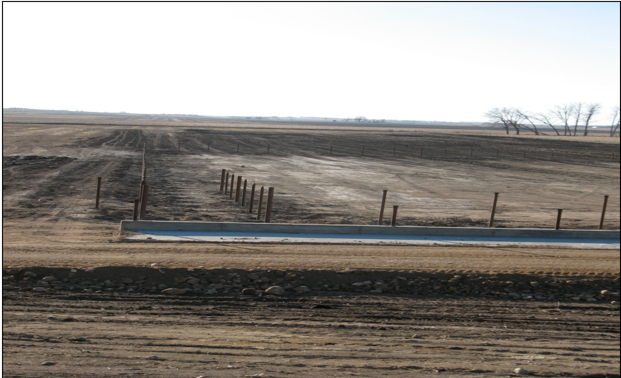
Figure 4: Newly constructed vegetative treatment area.
