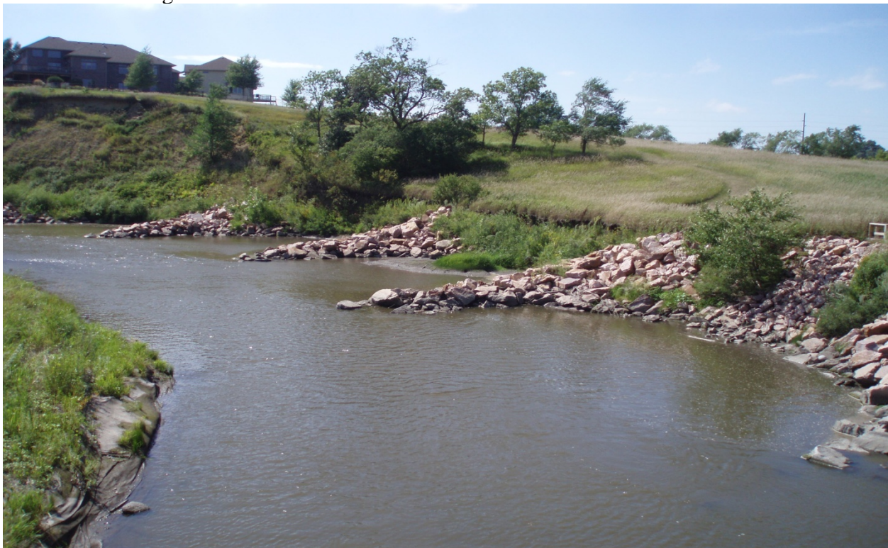
Figure 11: Skunk Creek bank stabilization and rock spurs.
