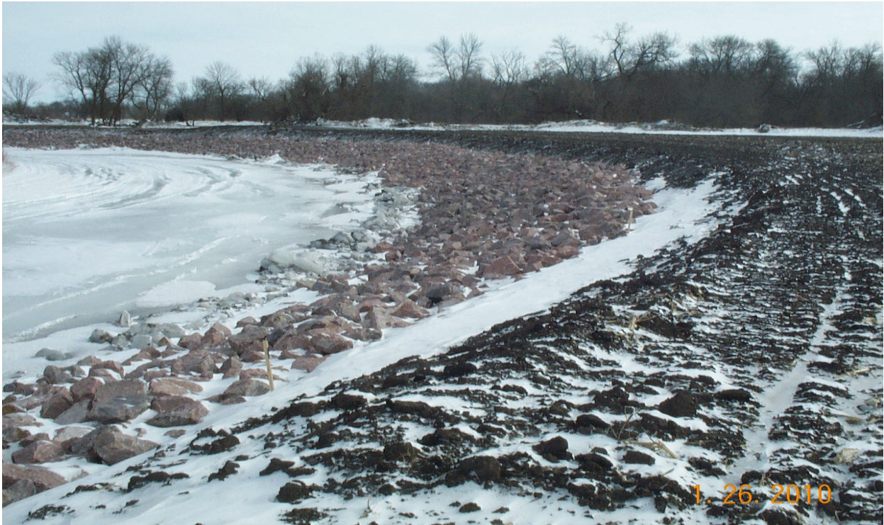
Figure 17: Segment 17 after placement of rip rap during the winter of 2010.
