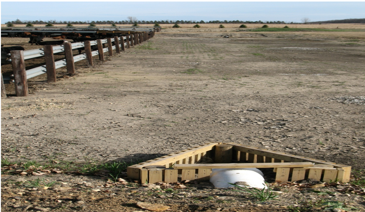
Figure 3: Feedlot Sediment Basin.
