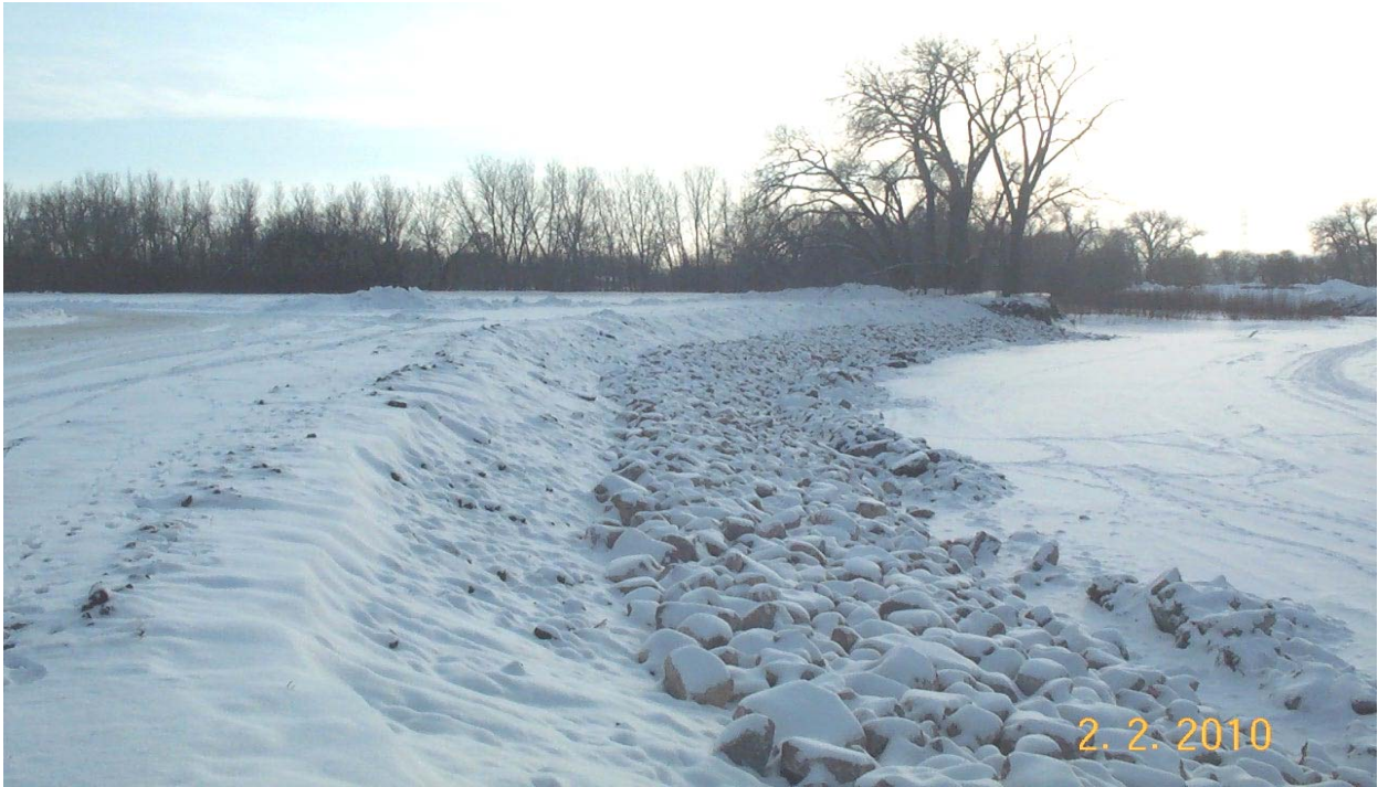
Figure 15: Rip rap placed on segment 65.
